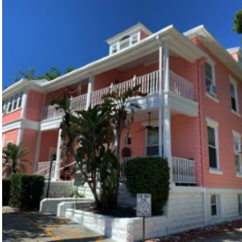
Vinoy Park Apartments At Beach Drive St Petersburg
